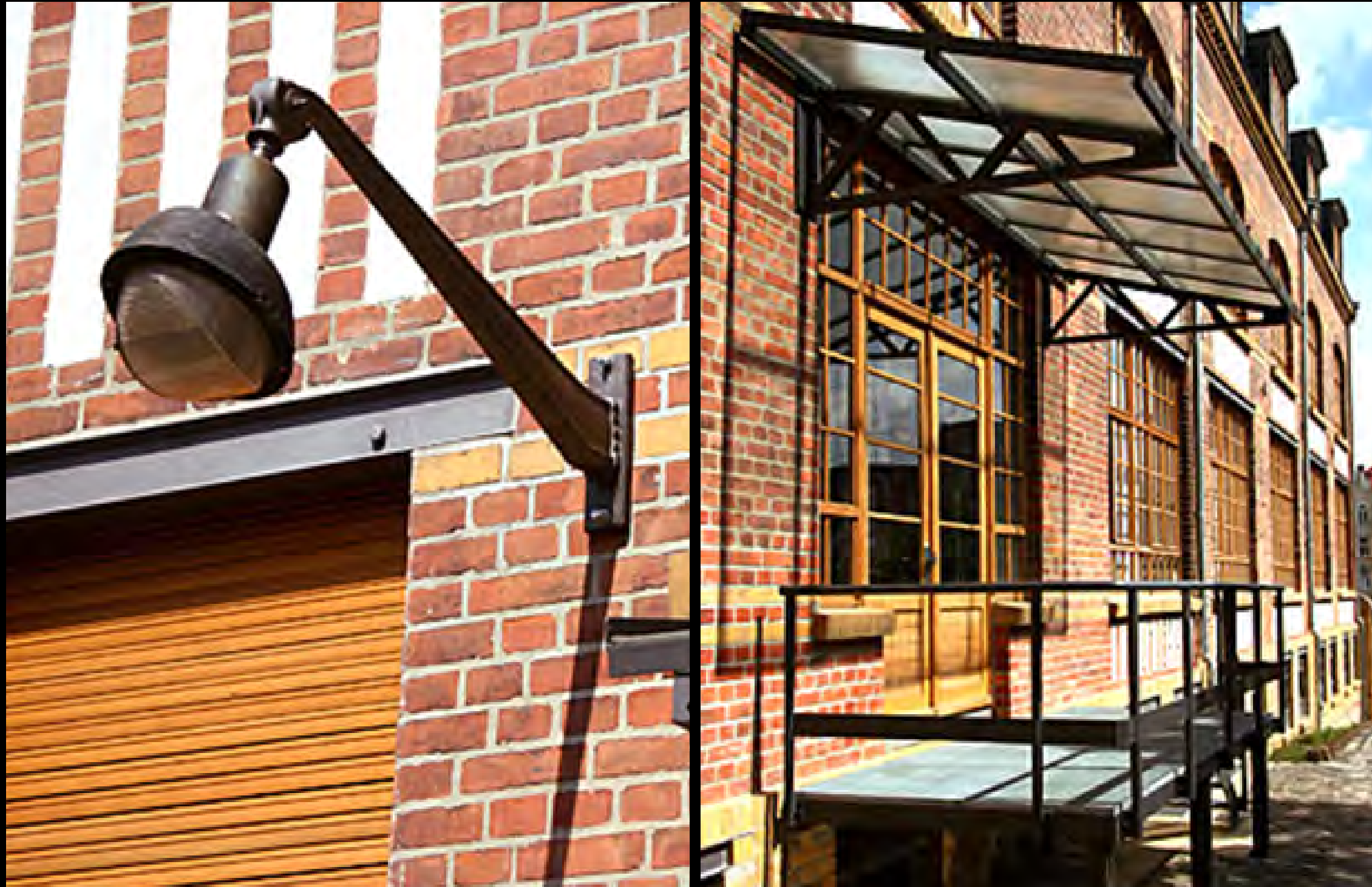
Details of the historical brick facade after restoration
