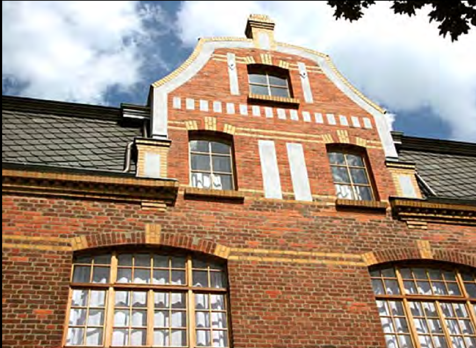
Gable view of the historical brick façade (Leipzig) after restoration
