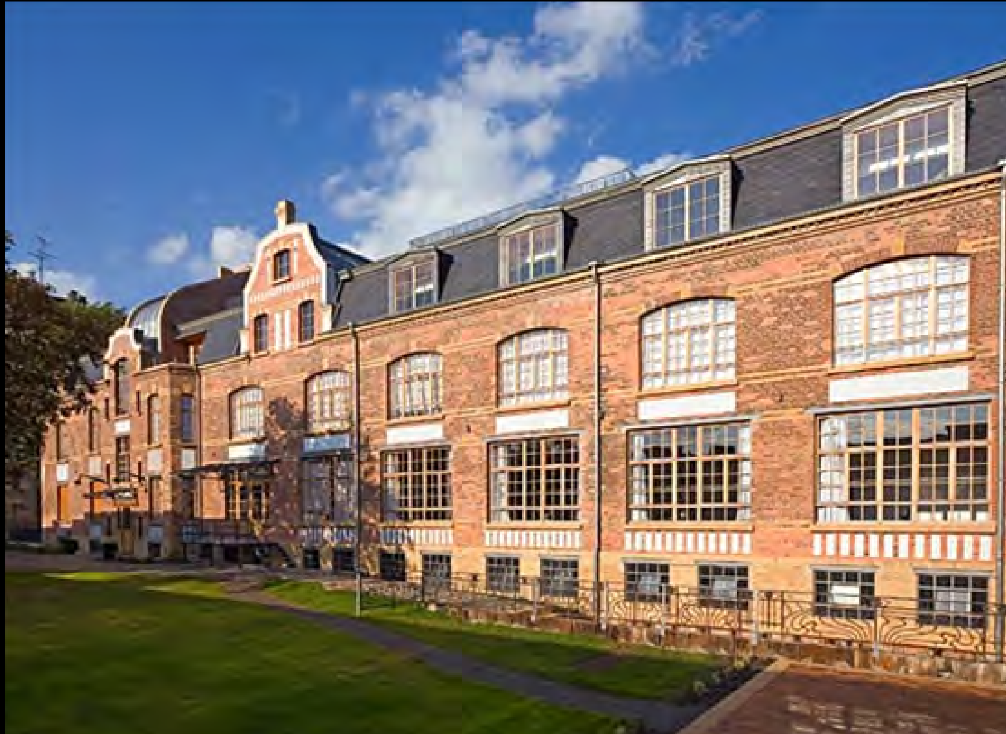
Factory Building from 1905 with historical brick façade (Leipzig), after restoration
