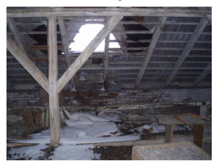
The roofing surface is not moisture-resistant. The apex is partially missing.
