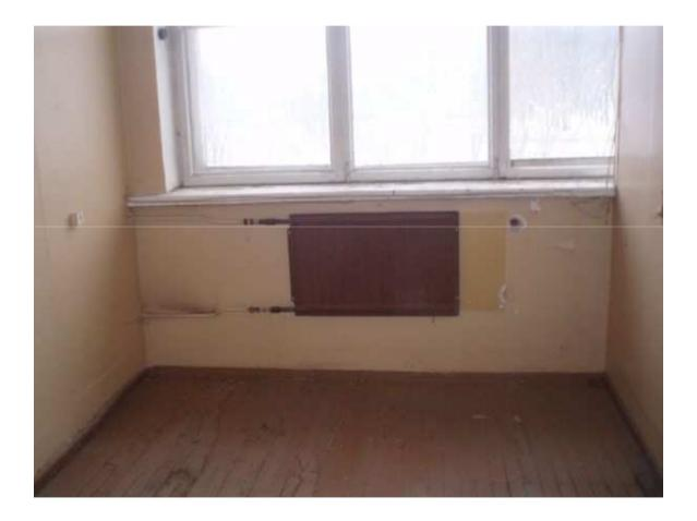
Some of the radiators are covered with decorative grating, which leads to lower heating efficiency.
