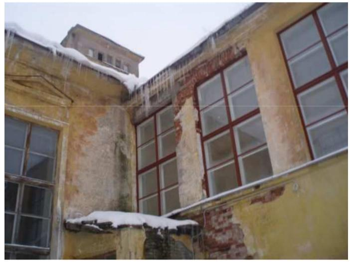
Moisture leaking through defective roofing combined with insufficient ventilation causes mould and structure disintegration
