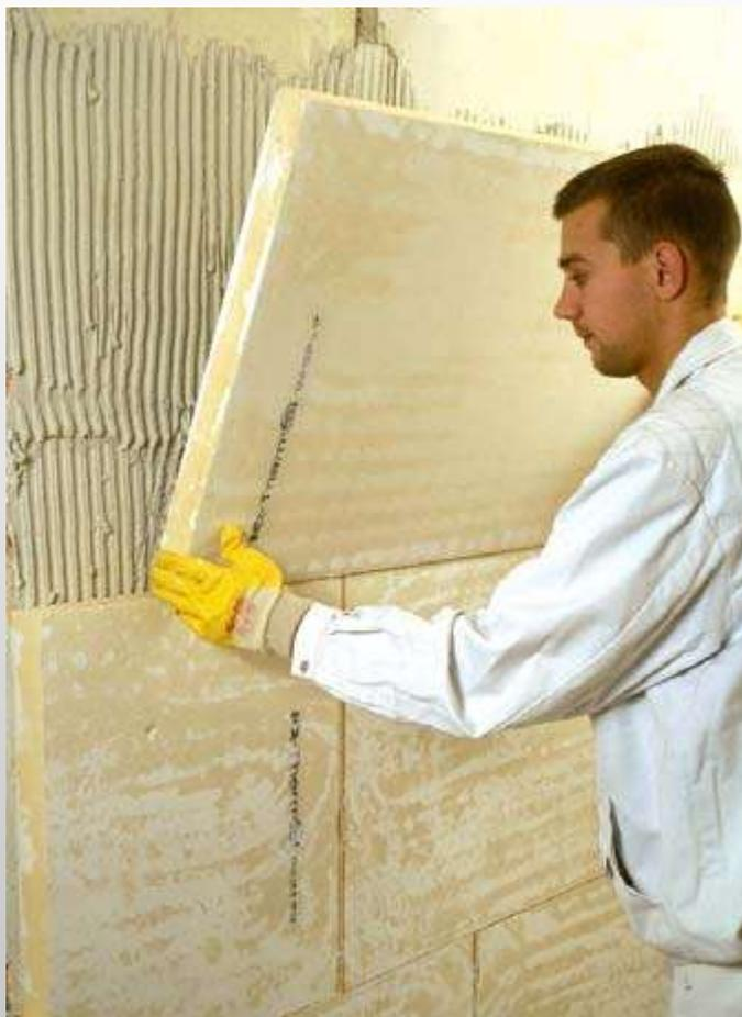
IQ thermal panels pressed into the fresh, the whole area coated any adhesive layer. Avoid cross stitches!
