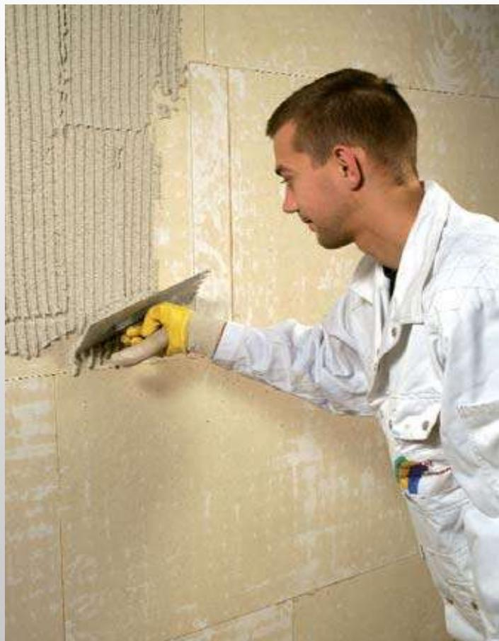
Top iQ is applied to a thermo as an upper mezzanine plaster layer. Thickness of about 5 mm notched.
