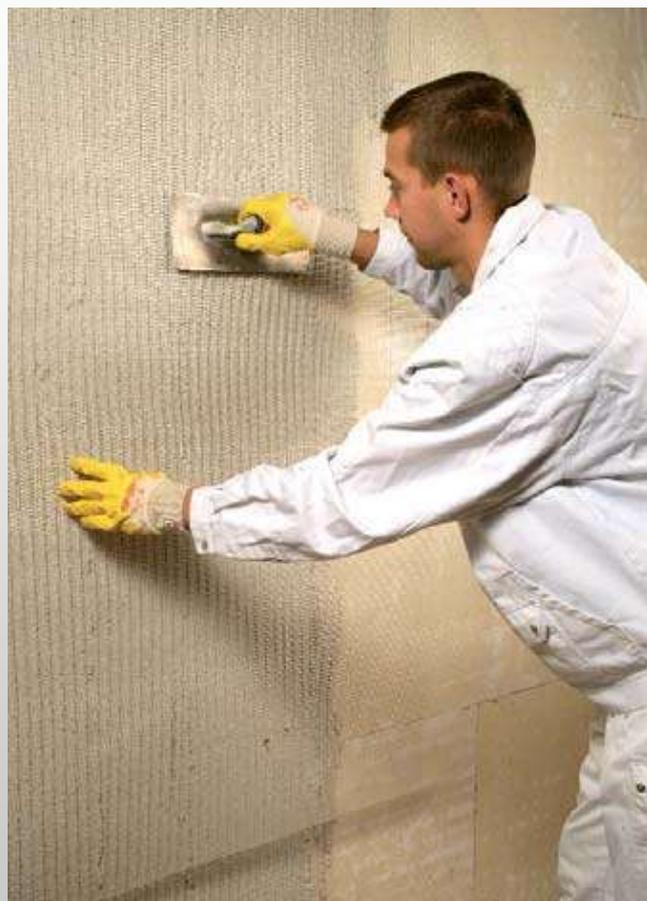
Mezzanine Tex fabric iQ mortar is applied to iron vertical stripes without wrinkles (separate fabric strips for at least 10 cm has come on top of each other).
