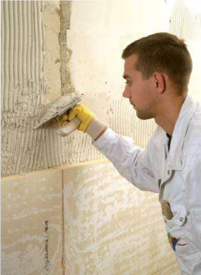
iQ Thermal panels attached the whole area to lock iQ (paste) high quality of the adhesive properties of the CIS marked by mortar intended iQ thermal plate bonding.
