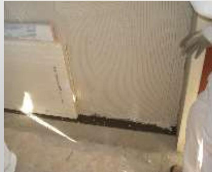
Glue on the wall spreads vertically (yield - 3.5 kg/m<sup>2</sup>), on a plate - horizontal (yield - 3.5 kg/m<sup>2</sup>). Apply glue equalized with comb.
