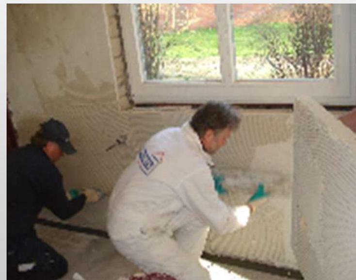
Where appropriate, in the IQ Thermo board are cutted out rips for heaters, sockets and cables. Shouldn't be butts in the corners of the window.
