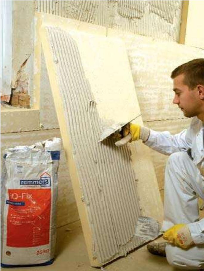
IQ lock on the level surface or plate of uniform covered with a toothed trowel (strips).
