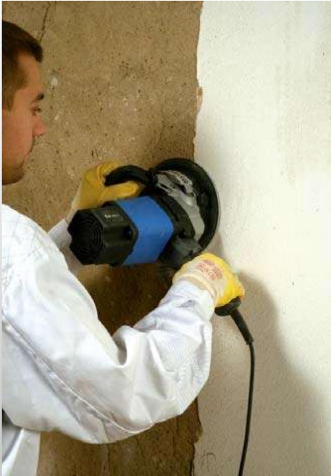
Removal of old paint by machines. The surface must be strong, strong enough on its not the individual particles or weak. Gypsum plaster filler should be removed. Very rough. The surface must be smooth and covered with plaster ground water, according to WTA technical description 2-9-04-D, in order to achieve complete system assembly.
