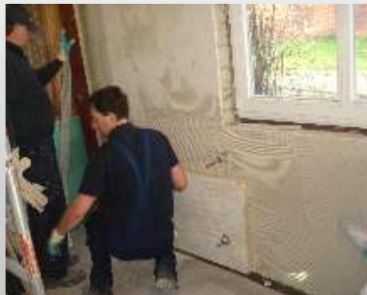
In working process windows must be plaster. The panels can be cutted in different ways, but corners must be refurbish. Windows inside and outside corners covered by a special angle fixer with the grid. Above the upper corners diagonally the extra grid has to be applied.
