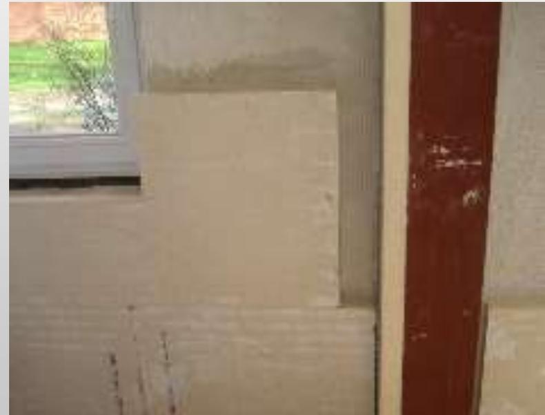
Finishing sticking process all the spaces are filled with polyurethane foam Pistolenschaum 1K. If on the other wall won't be iQ Therm plate, it is necessary to give the angle of the slope from 5 cm to 1 cm. Cupboard fittings are glued with polyurethane glue Coll Express Pu.
